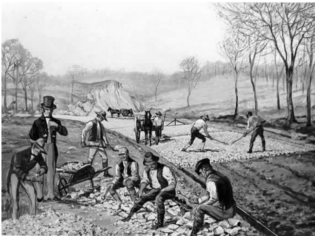
Workers laying macadamized roads.
